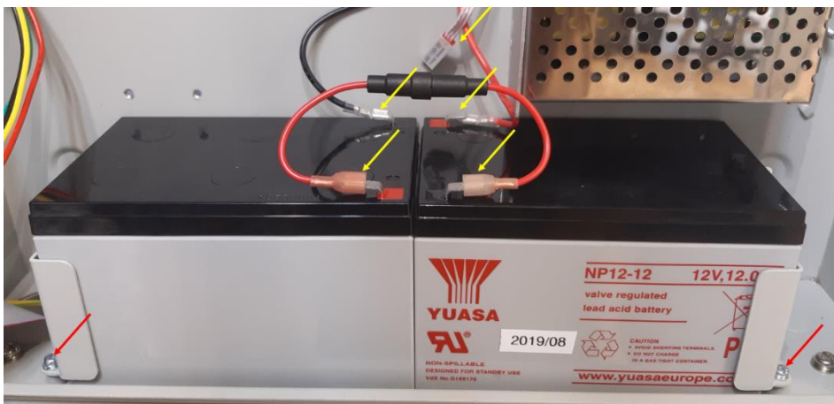
Figure 8: Battery Connection Locations for 7 & 12 Ah
