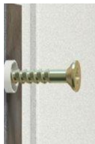
Figure 2: First screw for center keyhole
